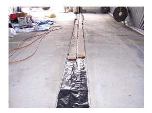
Over the top of the installed Moisture Seal, lay a plastic sheet to act as a bond breaker. Over the plastic sheet place plywood or cut lumber to apply a uniform pressure while the Tack Coat cures.
