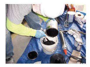
Combine & mix Part A & B of the Iso-Flex Tack Coat. The Tack Coat can be applied with a bulk gun or poured out and then spread with a margin trowel.
