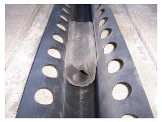
The Moisture Seal is held in place with sections of Iso-Flex Foamflux seal or properly sized backer rod. Be sure that 2.5" of the seal is on the blockout base and that the hole pattern will be fully sealed into the Tack Coat Material.
