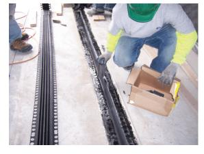
After 1-2 hours of cure, remove the foam seal or backer rod used to hold the Moisture Seal inplace.
