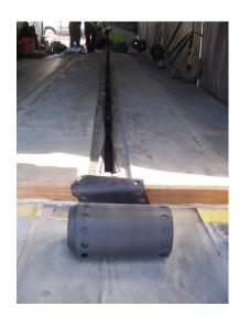
The process begins with rolls of the properly sized Iso-Flex Moisture Seal. This is a factory punched EPDM barrier.
